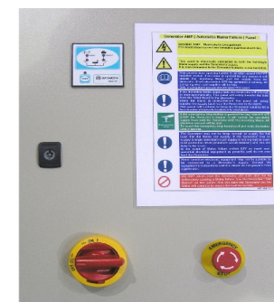
Typical Automatic Mains Failure Panel
